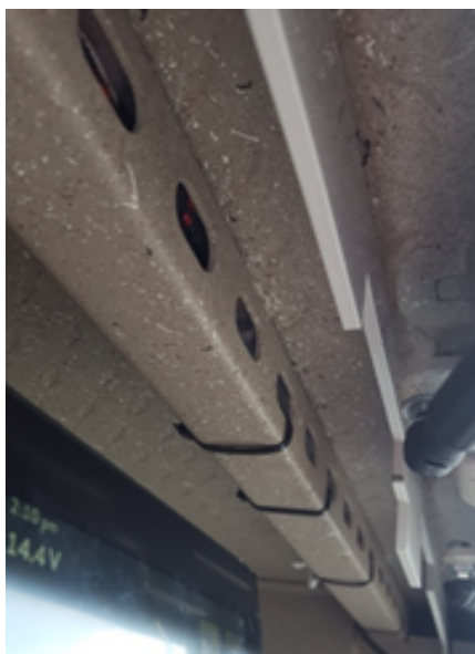
Figure 3 - Secure Channel Wiring
