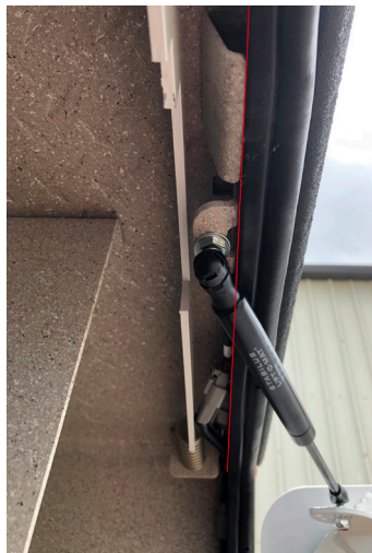
Figure 4 - Tall Compartment Wiring
